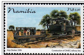
Construction of OMEG railway line
